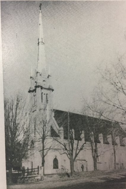
Exterior of St. Mary's after the turn of the century
